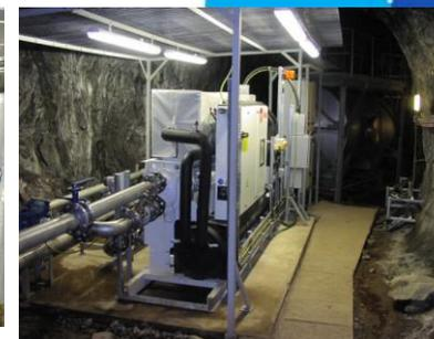
Following a Mott Macdonald survey and scheme design on behalf of Scottish Power, Nuvia were requested to tender for the detail design, installation and commissioning of a **new chilled water and buffer storage system** for the station. Nuvia approached JGC to partner with them on the project to provide MEC&I manufacturing, installation, testing and commissioning services. Following the competitive tender exercise, Nuvia and JGC were awarded the contract on **price and technical ability**.
